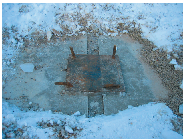
Figure 2.3. Anchor rods run over by crane.
