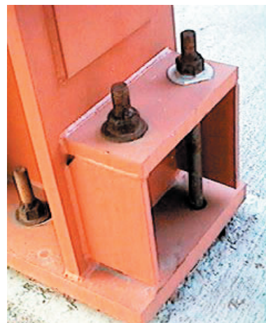
Figure A1.2. Column moment base using stool.
