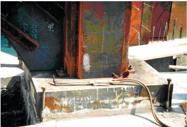
Figure 2.2. Base plate with adjusting screws.
