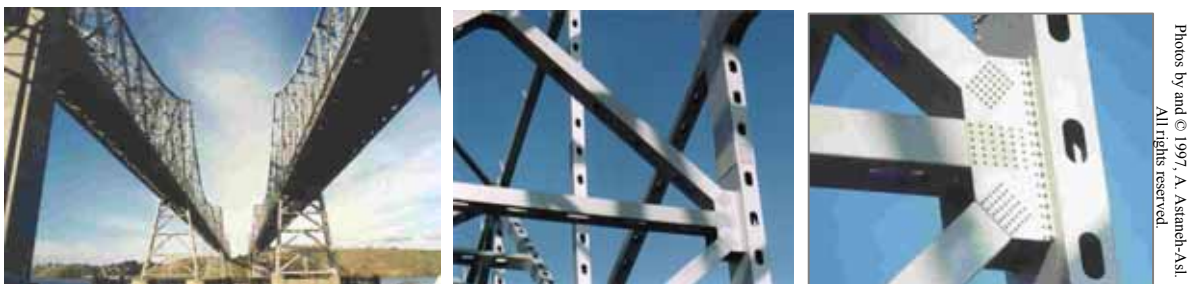
Figure 1.3. Double Gusset-Plate Connections of Carquinez Bridge Braced Frame Towers, Northern California
